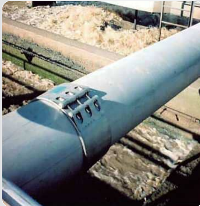
▶ Spanish water purification plant facilities
