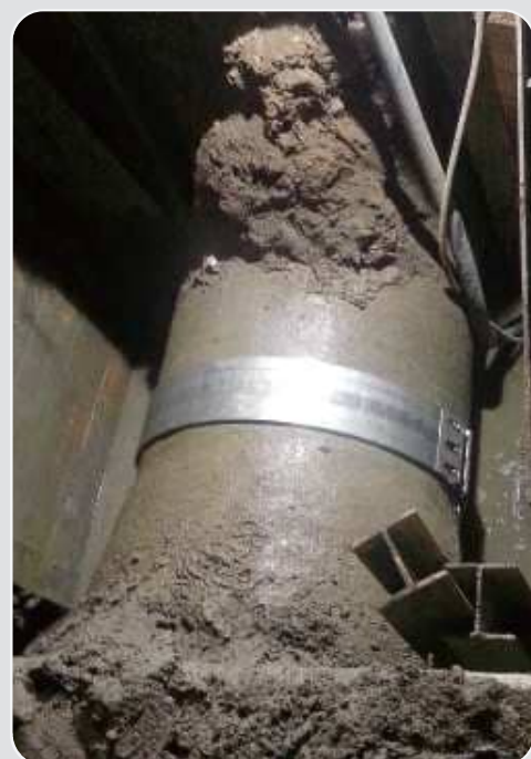
► Repair work on underground waterworks pipe line.
