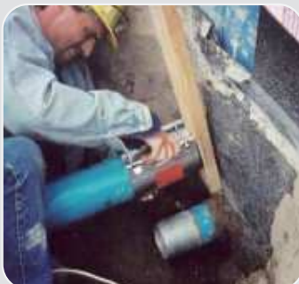
▶ Water and sewer maintenance work
