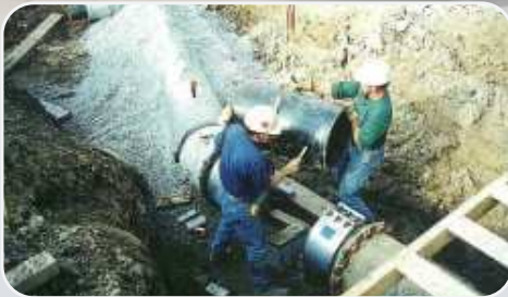
▶ Sewage Piping Repair Work
