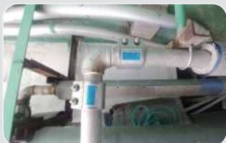
► Repair and installation of a corroded elbow line for an underground water tank.
