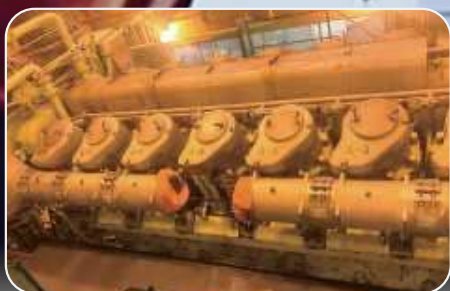
► Installation of emergency generator pipe systems for nuclear power plants.
