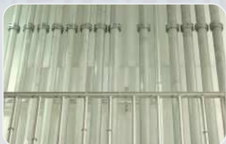
► Installation of a piping system for powder transport.
