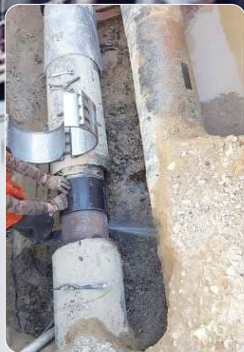
► Repair of piping for district heating power plants.
