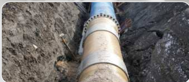
▶ Construction of Geumgang Boryeong Dam
