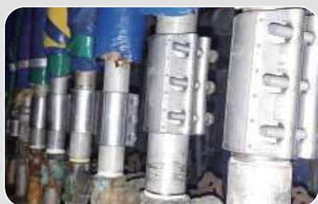
► Installation on underground pump pipes for apartment.
