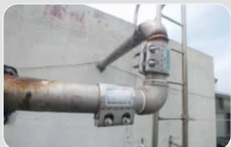
► Repair and installation of a corroded elbow line for an underground water tank.
