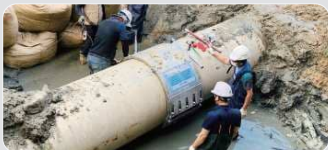
▶ Water repairing work of water fiber pipe
