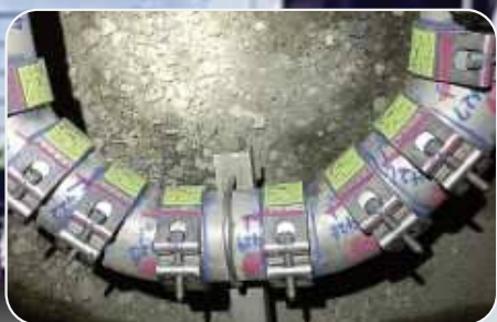
► Hydraulic pressure testing of clamps for repairing elbow pipes for Japanese railway bridges.
