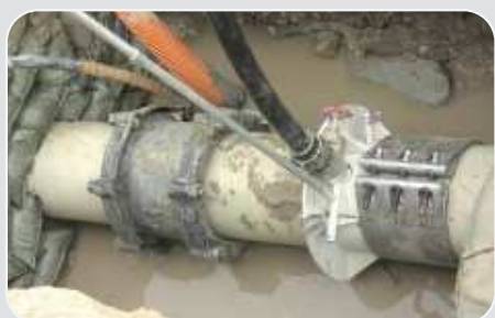
► Repair work on a 350A waterworks pipe line.
