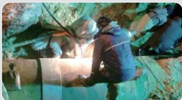
▶ Water pipeline leak repair work
