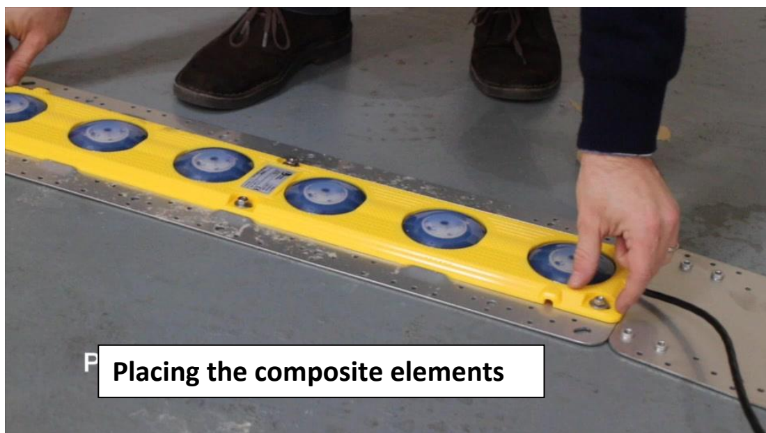
Figure 17 - Fasten the Composite Elements on the Lights
