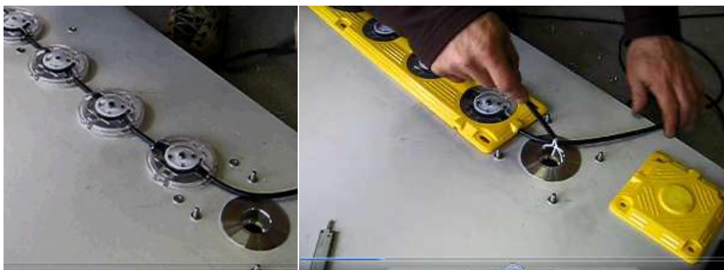
Figure 24 - Cables through Deck Installation
