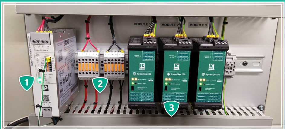
Figure 3 - The new ODS installation consisting of a galvanically isolated SELV power supply (1), a double 24V supply distribution for a possibility of redundancy (2), and three SpeedSys 200 units, hardwired to form a 2oo3 voting structure (3).
