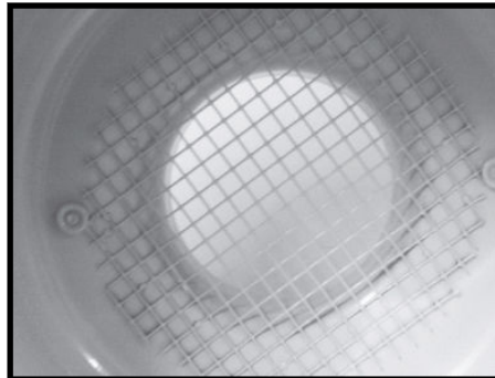
Step 8. Check inlet grille is clear.
