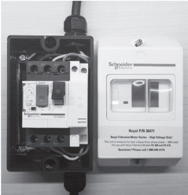
Figure 1. The visual appearance of the starter/isolator, showing internal (left) and external (right) views.
