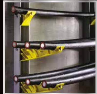
BNT Saddle Arms Installed in a Nonmetallic Stanchion
