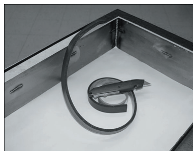
3.27. Installation of Top Cover Seal
