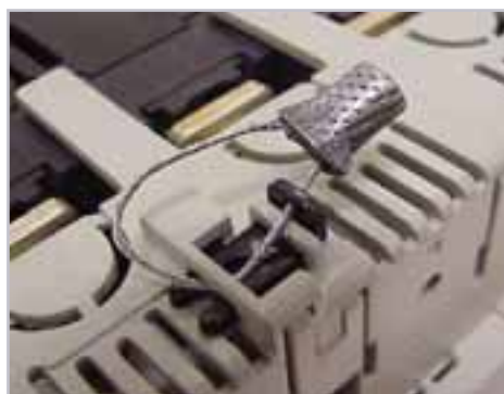
Terminal Cover Lock with Lead Seal
